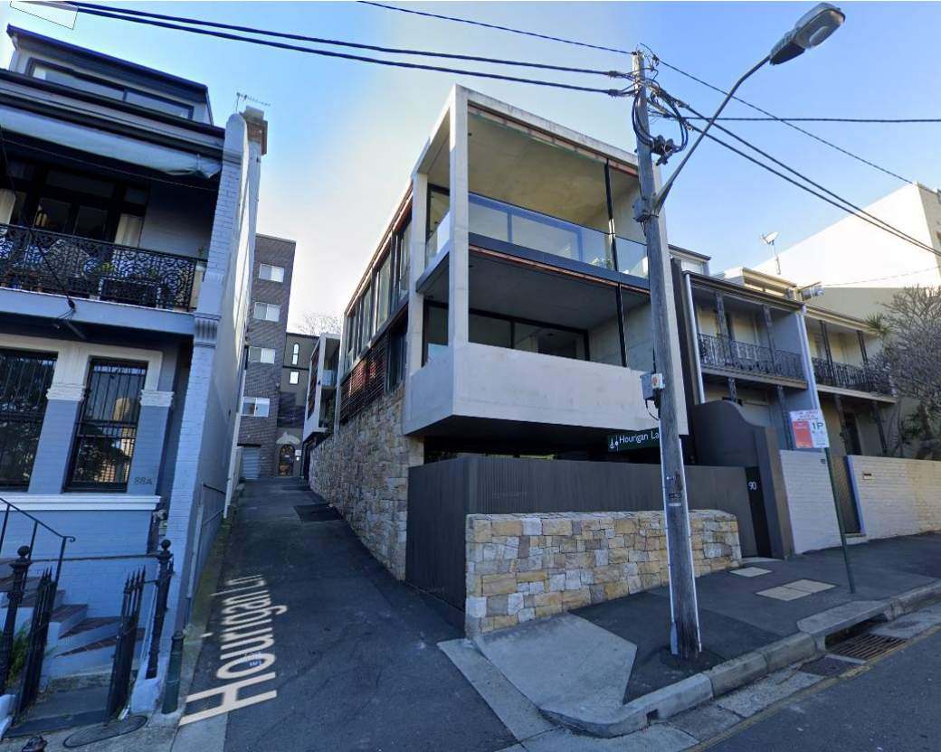
Figure 2. 90 Brougham Street looking east from Brougham Street
